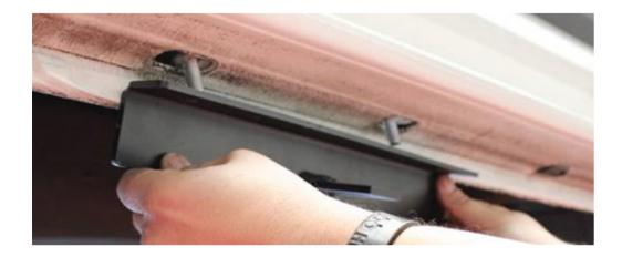
For the middle brackets, remove 2 caps an place boldplates and connect the bracket.
